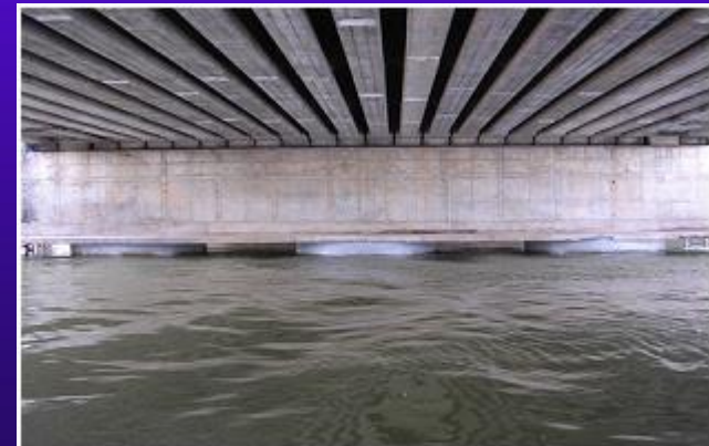
5. After GFRP application
