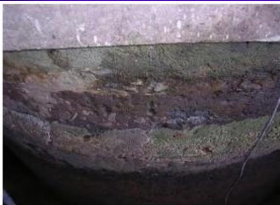
3. Scaling and cracks
