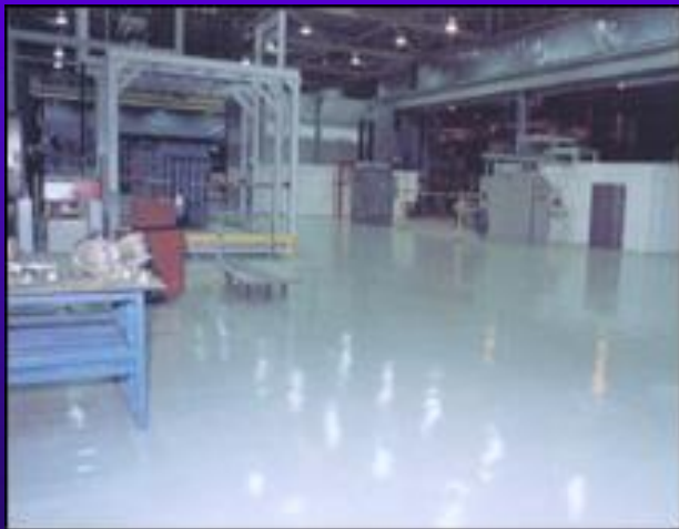
Prime Floor and Topcoat
