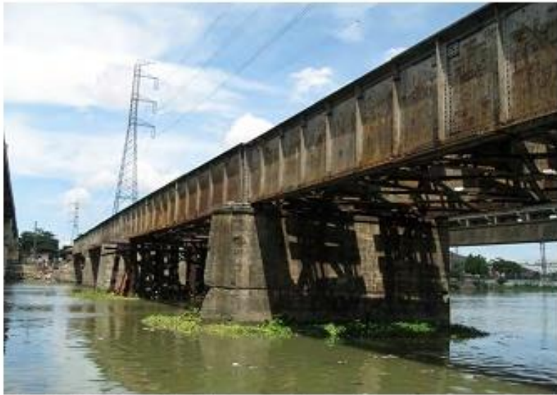
1. Railway bridges without maintenance
