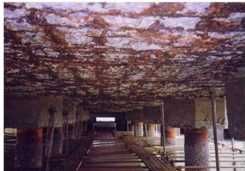
2. Rebar corrosion
