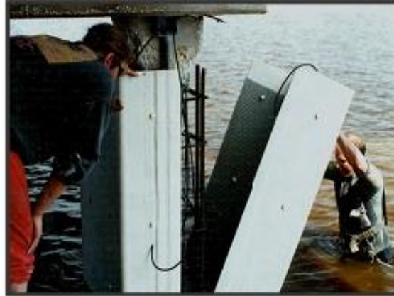
Rebar & FRP Form Installation
