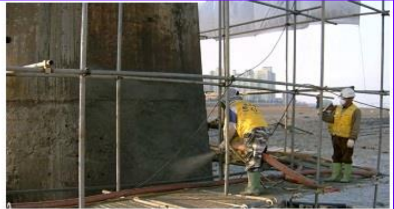
2. Dry Shotcrete application
