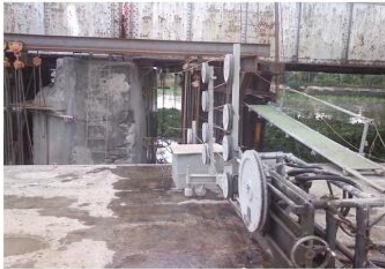
3. Wire-saw underwater cutting
