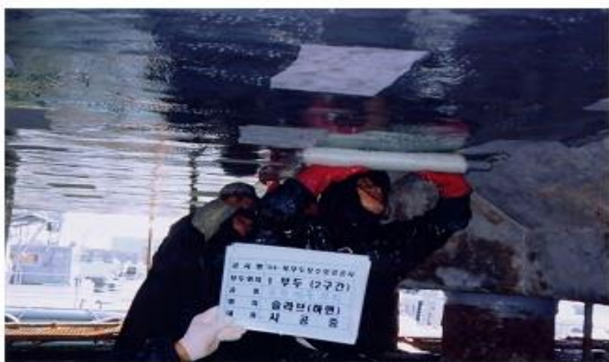
3. Strengthening with GFRP
