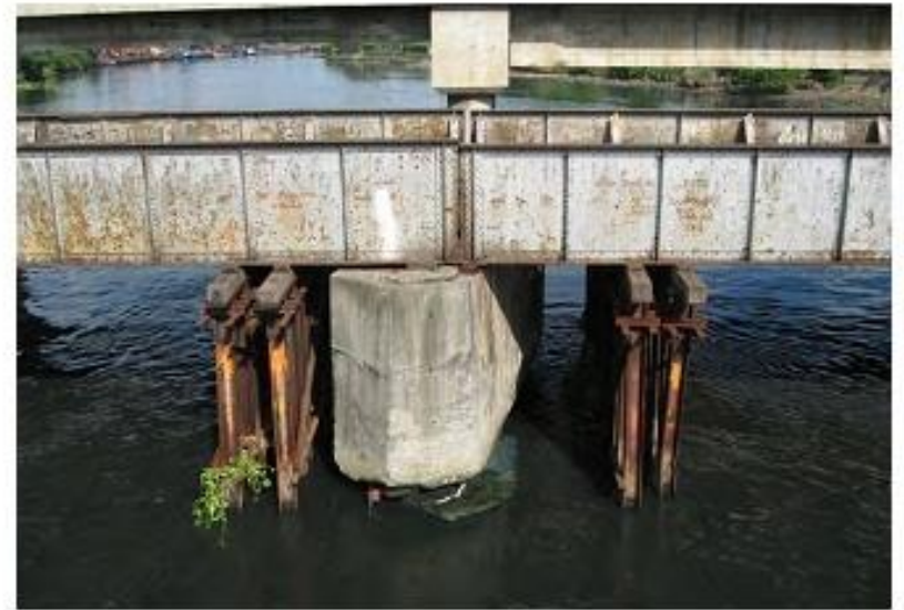
2. Pier #2 was broken by ship
