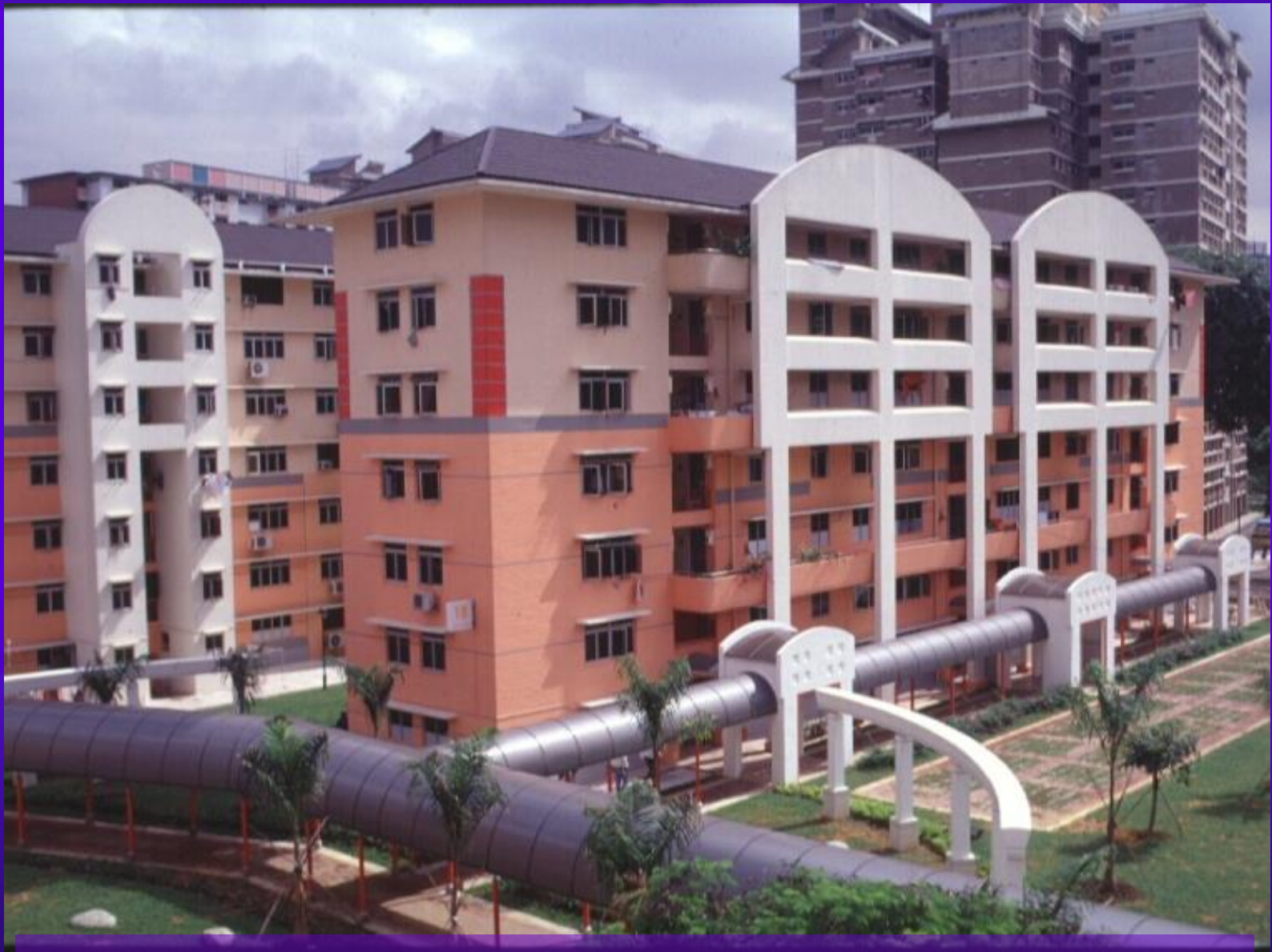
New appearance of a typical block after upgrading
