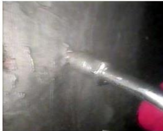
5. Injection UW epoxy
