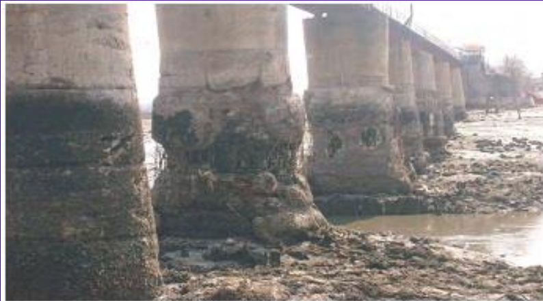
1. Erosion and corrosion problems
